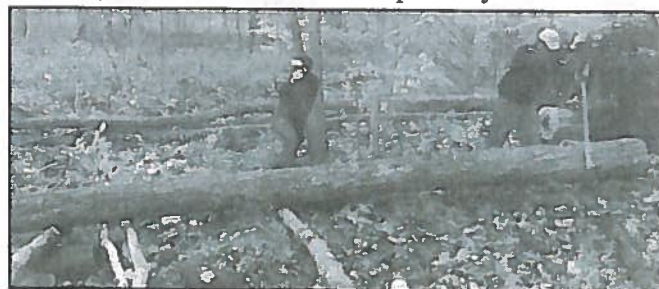
Bridge building on North Boundary Trail
